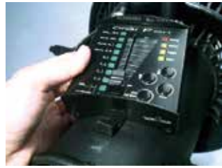
Switch for local or DMX operation mode.
